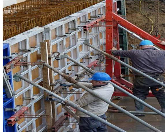
Shuttering and RCC casting coordination around pipe penetration.
