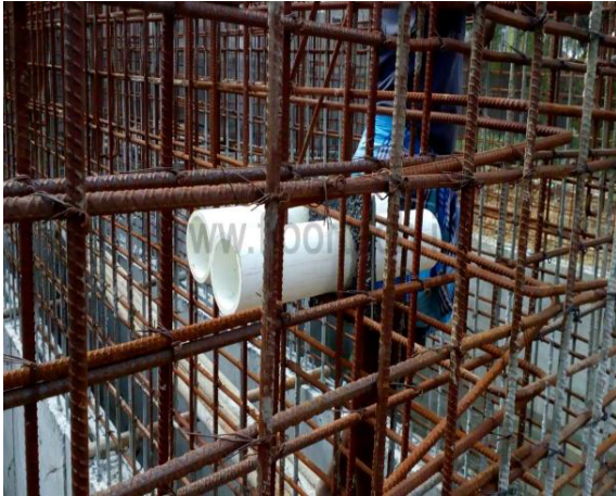
Puddle flange positioned with reinforcement before concreting.
